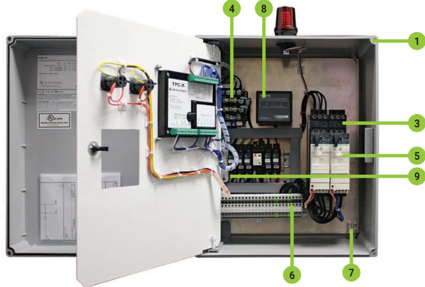
The Model 32XR control panel is designed to alternately control two three phase pumps in industrial and commercial water and sewage systems using a 4-20 mA level transmitter. In addition to transmitter control, this system will accept a high water float to activate the alarm and run both pumps. This panel also provides a redundant low level cutout, seal fail and thermal cutout for both pumps. Common applications include lift stations, pump chambers and irrigation systems.
